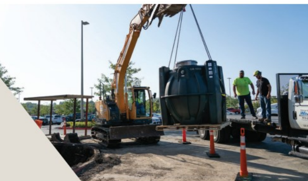
▲ GB-1000 Installation - Costco
