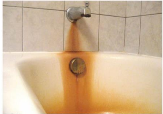
Image of iron staining.
