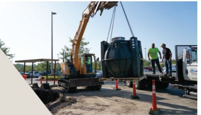
▲ GB-1000 Installation - Costco
