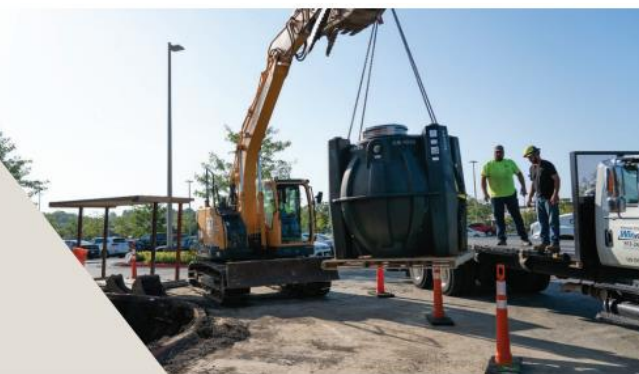
▲ GB-1000 Installation - Costco
