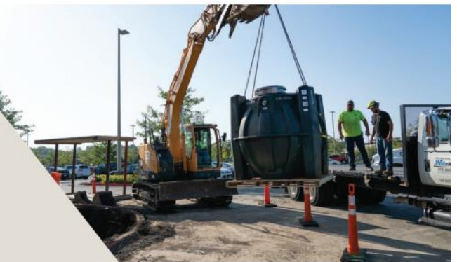
▲ GB-1000 Installation - Costco
