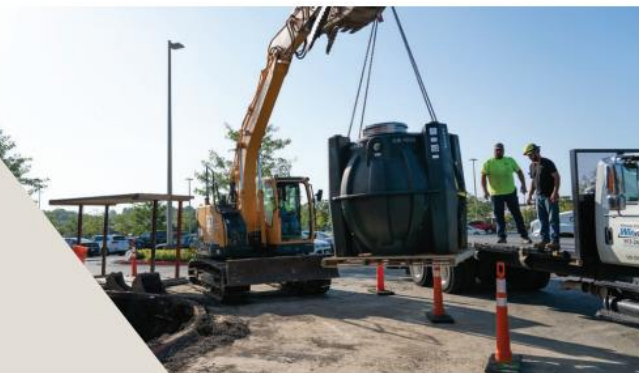
▲ GB-1000 Installation - Costco
